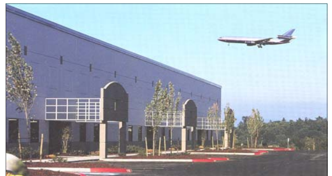
Premier Airfreight Facility in Seattle
